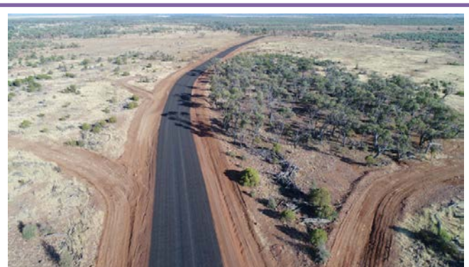
Strathroy Road (Jump up) Upgrades – May 2018
