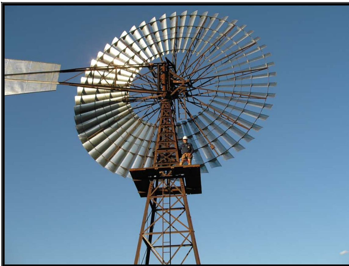
35 FT WINDMILL BEING ERECTED RIVERSIDE PARK
